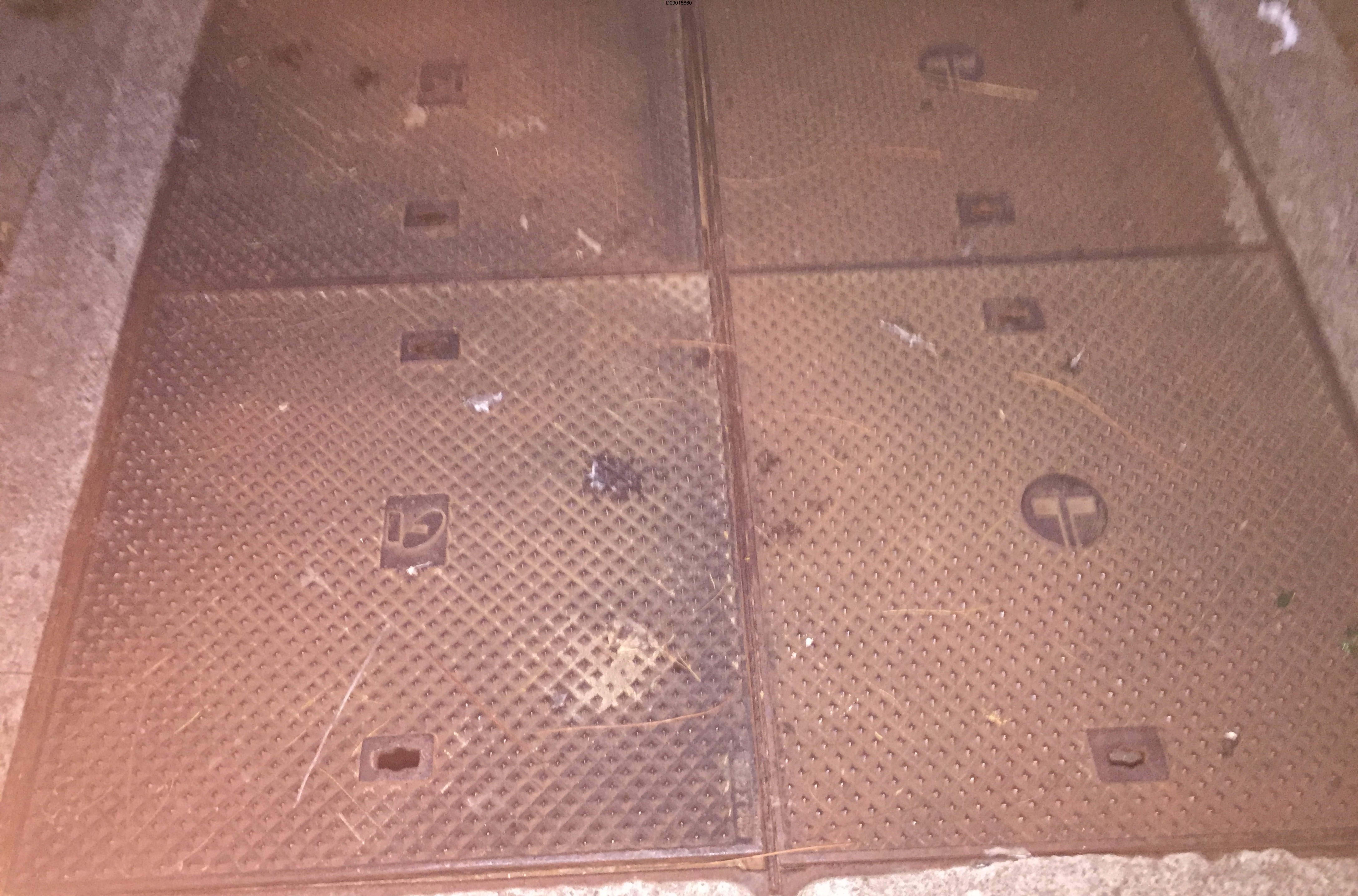
PHOTO TAKEN 12/07/18 SHOWING LARGE TELSTRA TELECOMMUNICATION PIT LOCATED ON THE CORNER OF BAY STREET & ARNOTT AVENUE
